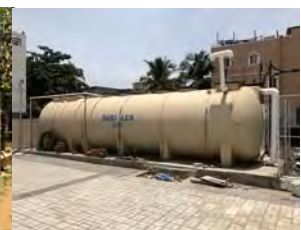
COMMERCIAL BUILDING (40KLD)
